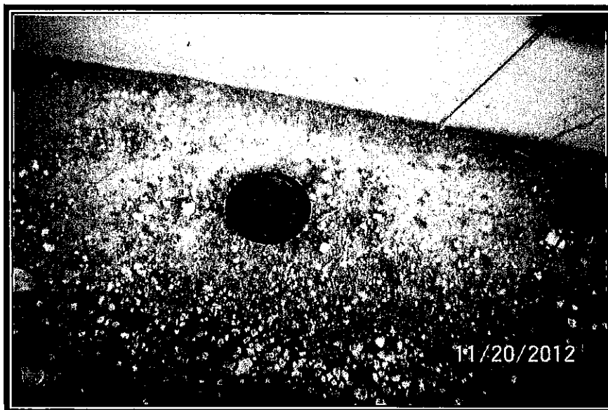
TERMITE CONTROL ON EXTERIOR OF IMPROVEMENT
