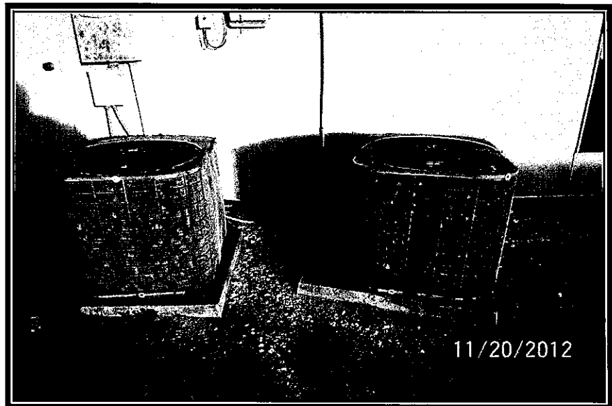
DAMAGED HVAC UNITS
